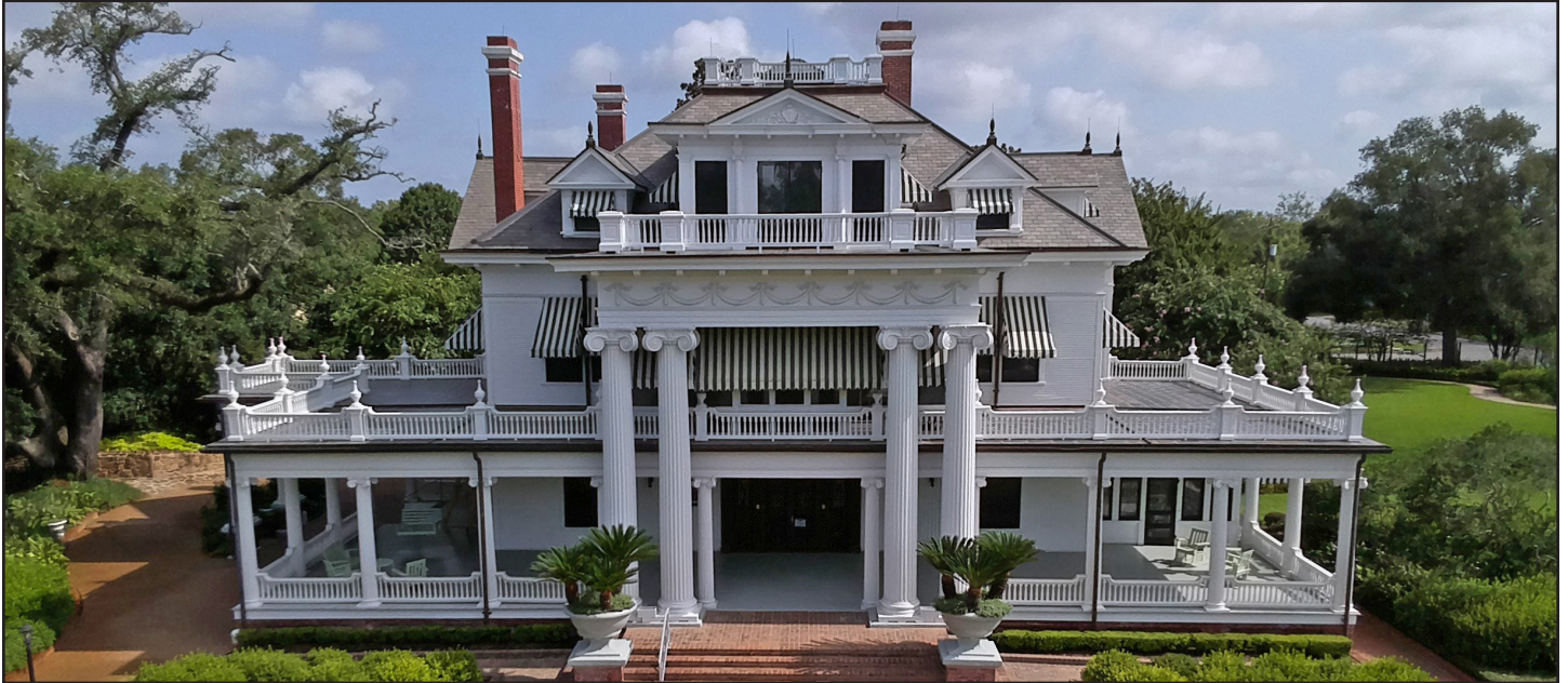
The McFaddin-Ward House was designed with architectural features such as spacious porches, transom windows, and tall ceilings to help with cooling.
