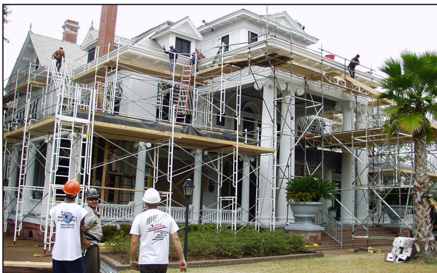
Oak Grove led the roof restoration project in 2001.
