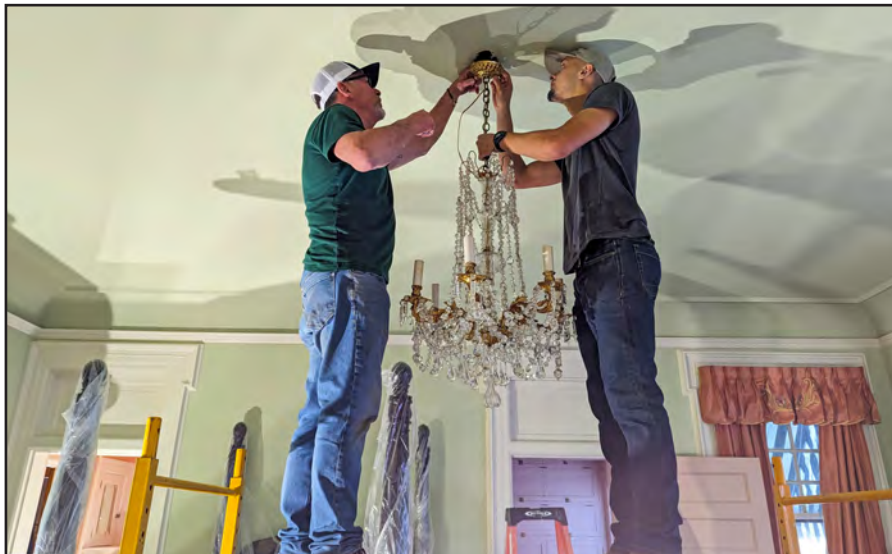
Oak Grove Restoration Co. removes the chandelier in the Primary Bedroom for rewiring.
